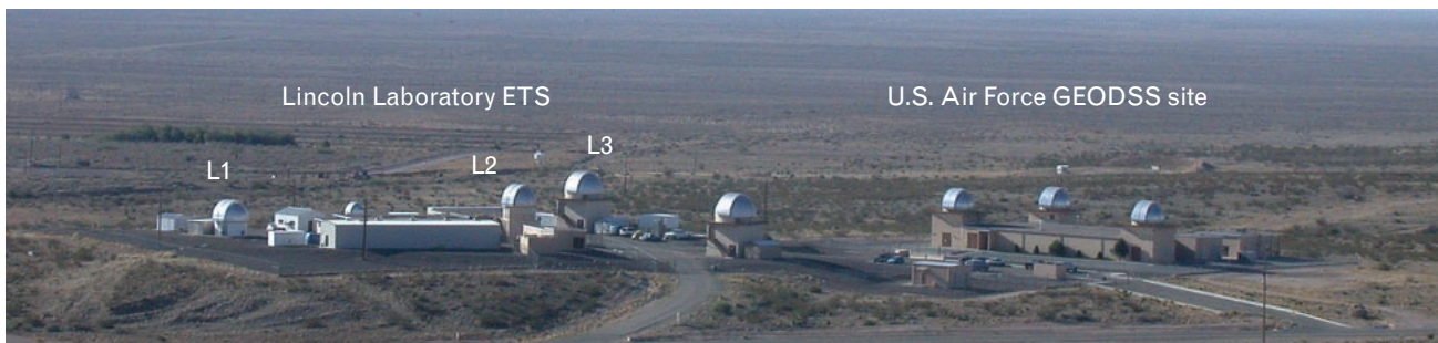
FIGURE 3. The ETS at White Sands Missile Range, near Socorro, New Mexico, adjacent to the U.S. Air Force GEODSS site. The LINEAR program operates two search telescopes, called L1 and L2, and one follow-up telescope, called L3.
