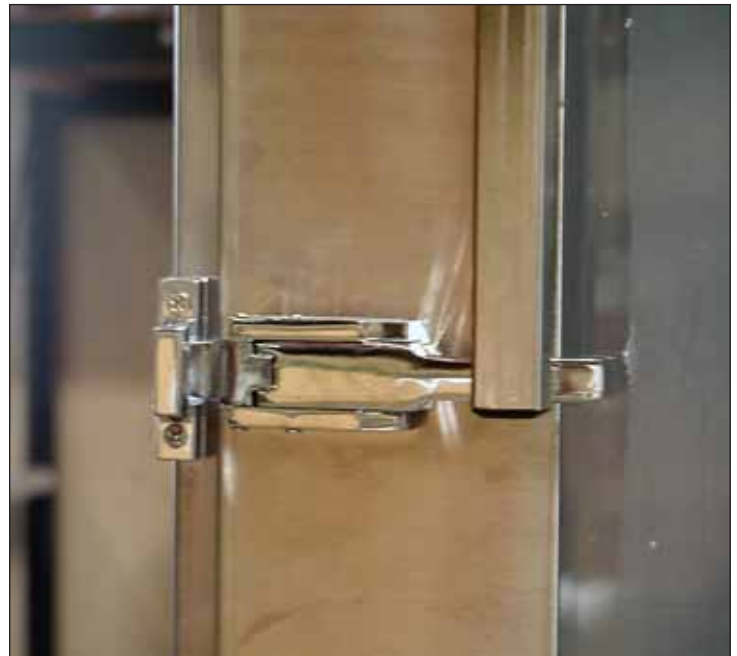
Door Latch Correctly Centered
